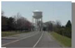
Water Tower Replacement
