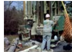
Refurbishment to lift stations
