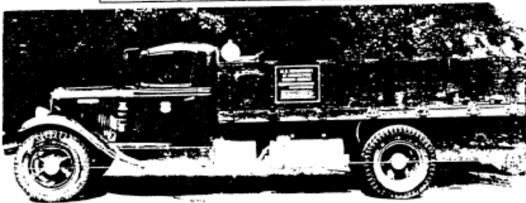
Figure 6.--Gasogen mounted on FPL truck--1942.
