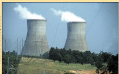
Cooling towers, Burke County, Georgia
