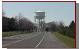
Water Tower Replacement
