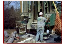
Refurbishment to lift stations
