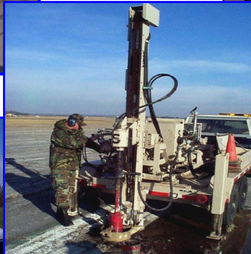
CORE DRILL (Structural)
