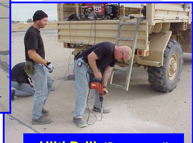
Hilti Drill (Structural)
