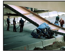
Denver highway beam
