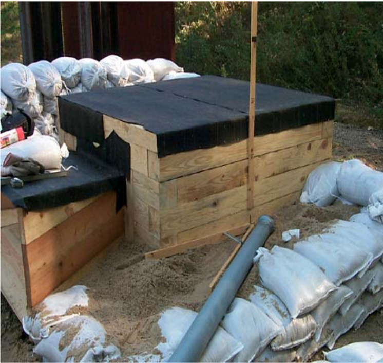
6" x 6" side timbers 4" x 4" top timbers
