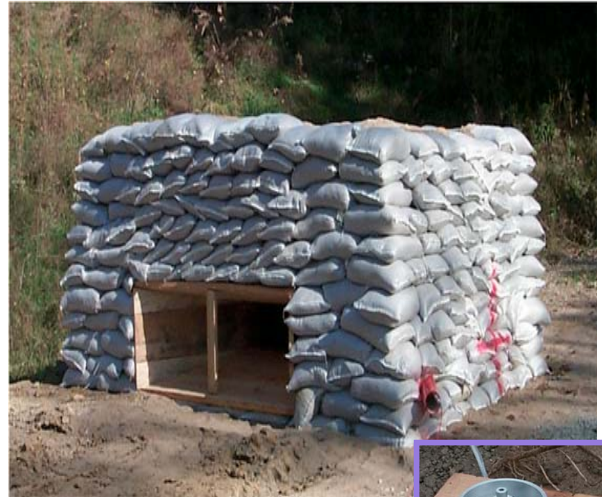
3' thick sand wall with interlocking sand bags
