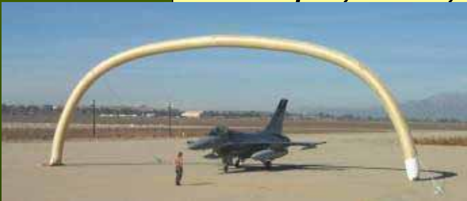
82 foot span, 30" dia, 80 psi
