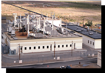
Infrastructure in place with state-of-the-art equipment
