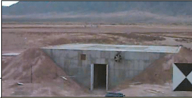
One of several identical test structures
